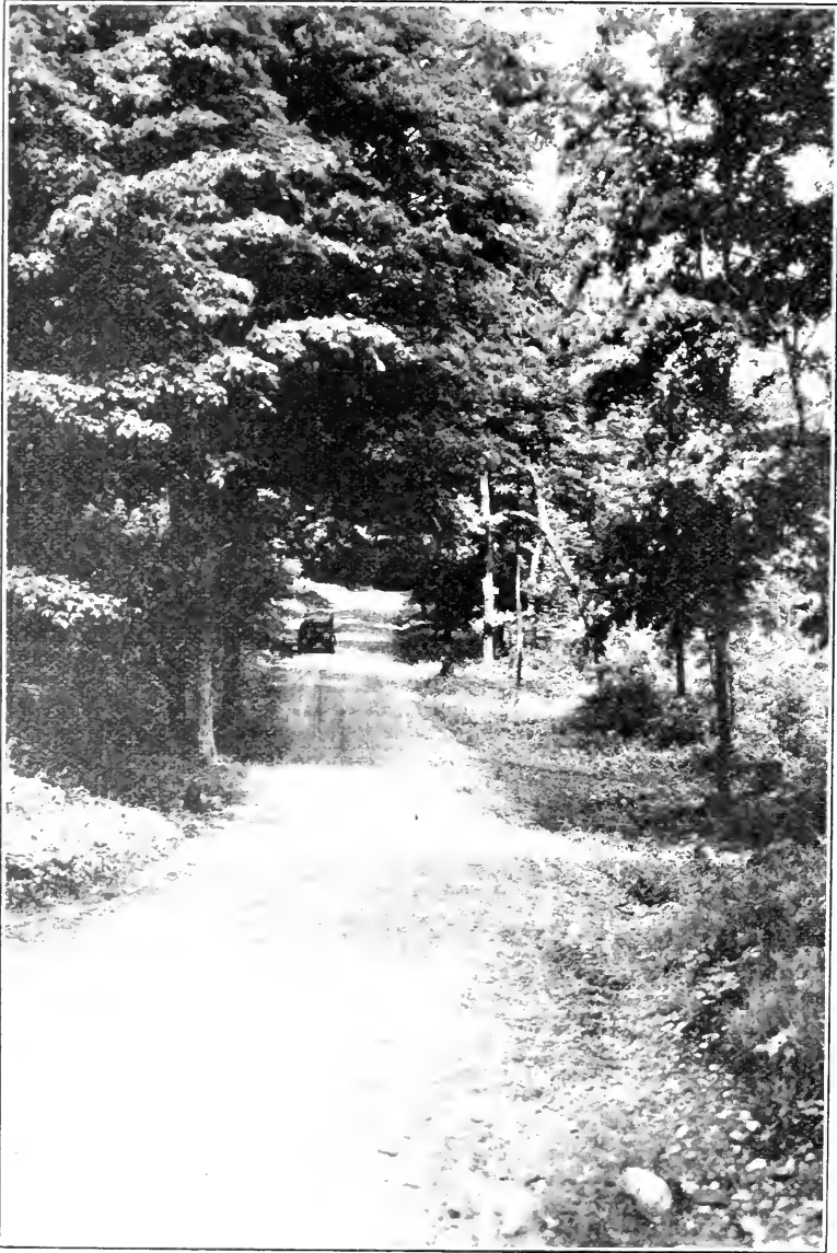
Ferguson Highway—South of South River.
